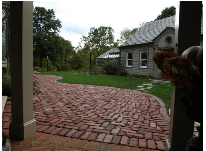
Curved sidewalk of street brick pavers installed in herringbone pattern.
