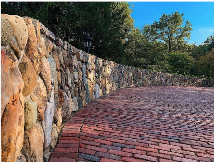
Entrance parking pad of reclaimed bricks next to stone wall.
