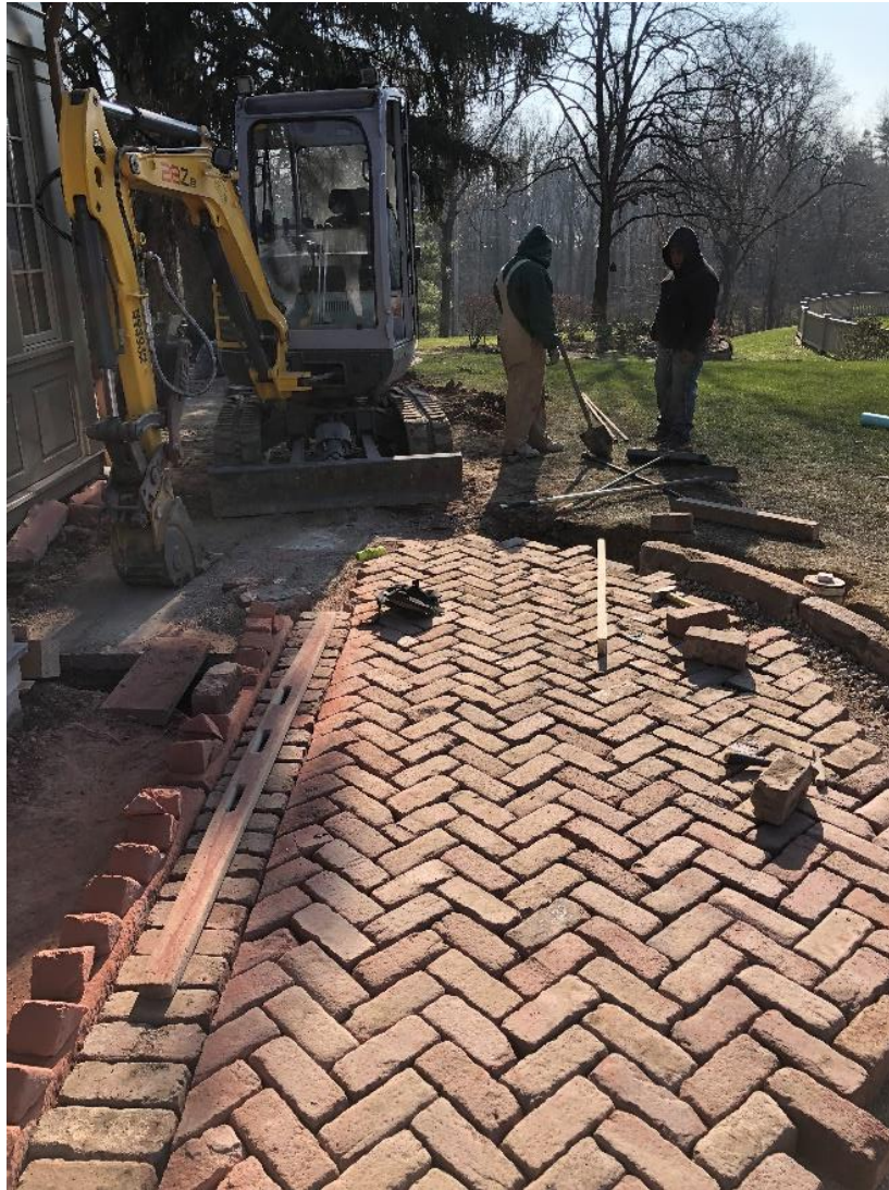
Construction begins, street brick pavers installed in a herringbone pattern.
