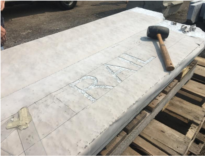
Prepping the granite curb for the project engravings.
