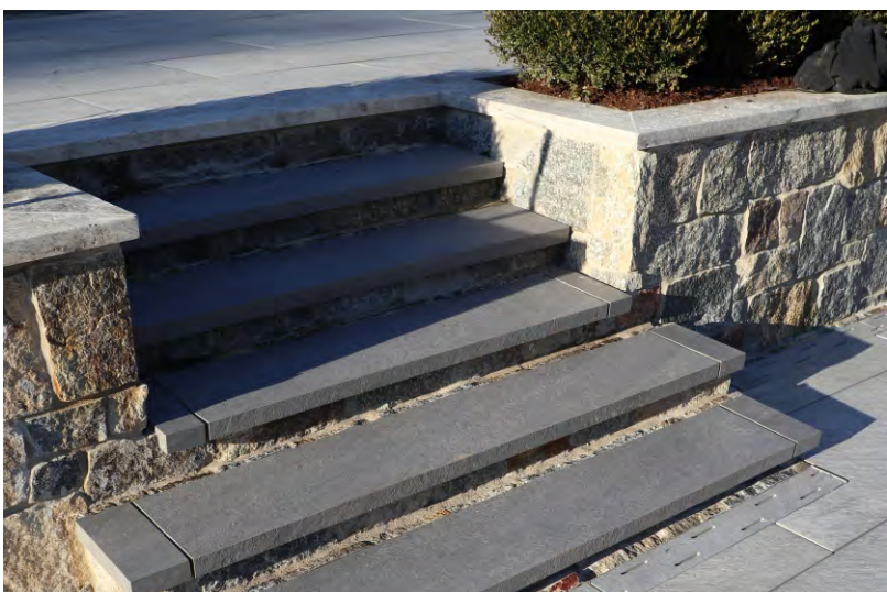
Mitered steps and custom drains
