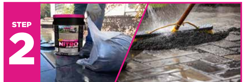
Spread, wet and fill joints with Gator Nitro Sand.
