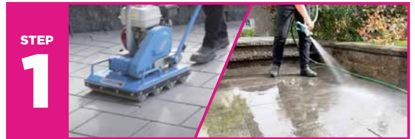
Compact first, then wet the paved surface.
