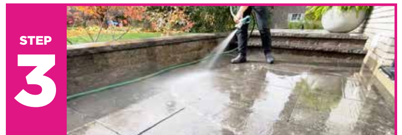
Remove all excess Gator Nitro Sand by rinsing and brushing until the entire paved surface is clean. Please read our TDS (visit AllianceGator.com) for the complete installation steps.
